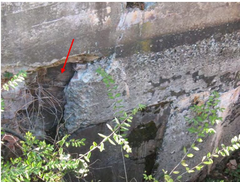
Photo 14. Hunt's Mill Dam. Concrete deterioration of riverside headrace open flume wall. Note stone masonry exposed due to missing concrete cover (arrow).
