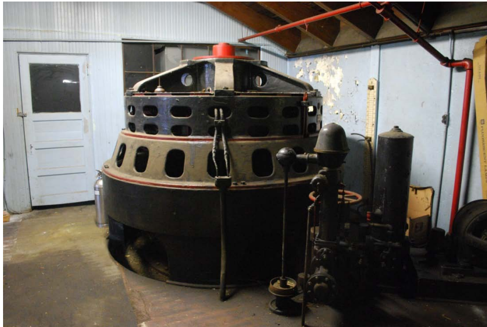
Figure 4. Existing Hunt's Mill Generator and Governor
