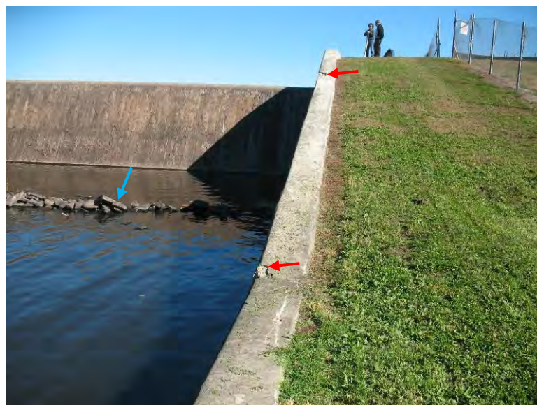
Photo 3. Turner Reservoir Dam. Left retaining wall. Note areas with concrete deterioration (red arrows) and pile of stone in tailwater (blue arrow).
