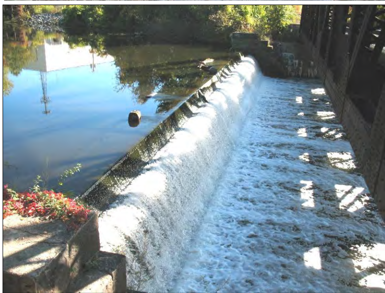
Photo 17. Omega Pond Dam. Spillway and left abutment.
