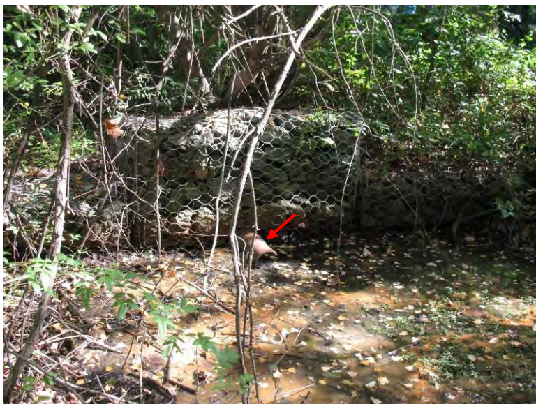
Photo 6. Turner Reservoir Dam. Stone gabion wall with drain pipe outlet (arrow) at toe of left embankment.
