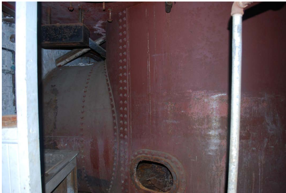
Figure 5. Steel penstock and Vertical Pressure Case
